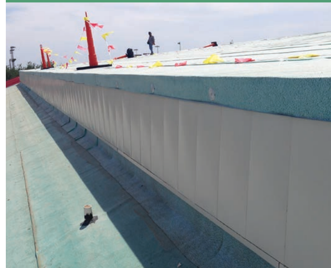
All the metal panels for the project were formed on-site by Rio Roofing craftsmen.
