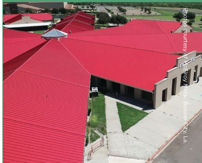
Rio Roofing workers fastened 141,800 lineal feet of McElroy Metal symmetrical standing-seam Galvalume® panels in PVDF Brite Red.
