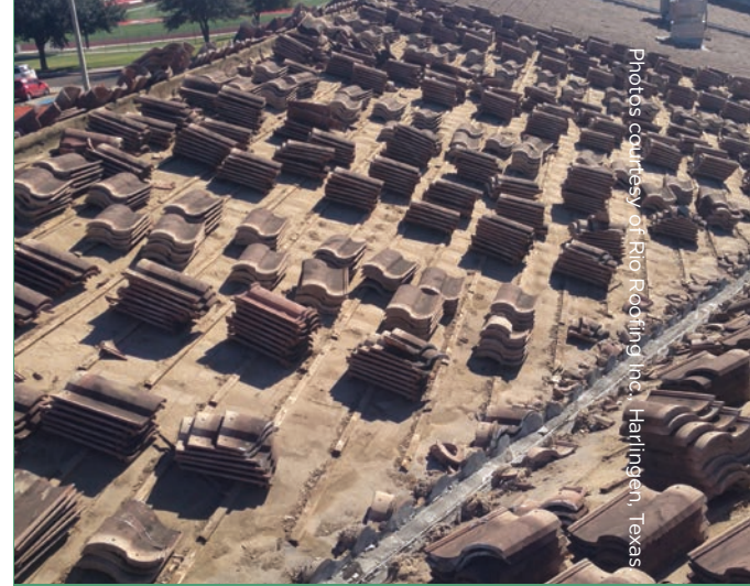
Rio Roofing workers removed the existing tiles from the 190,000-square-foot main roof areas.
