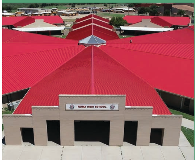
An aerial view of Roma High School's new metal roof system
