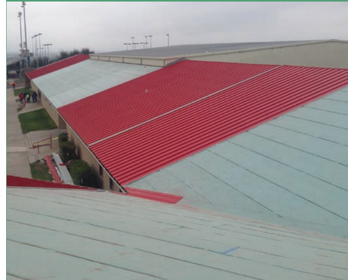
All the metal panels for the project were formed on-site by Rio Roofing craftsmen.
